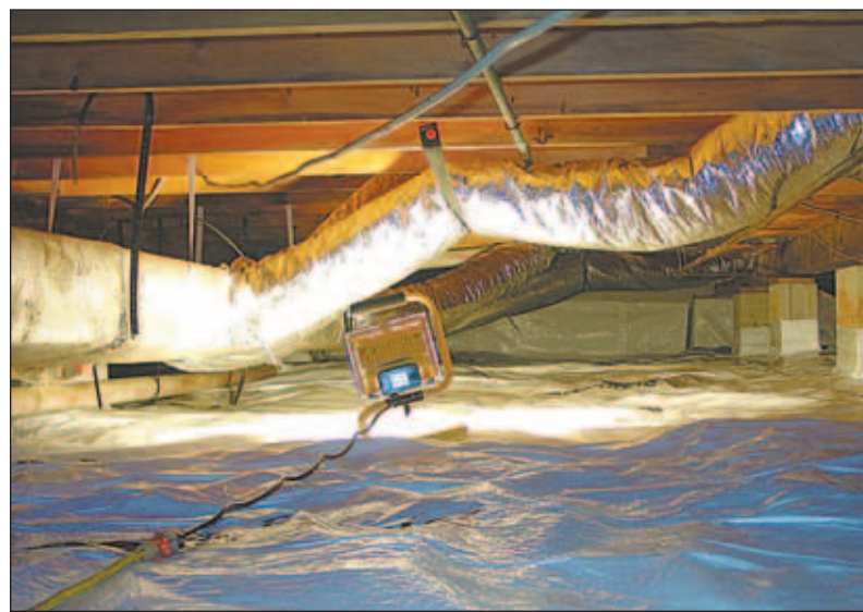
ABOVE Before. BELOW After. Encapsulation of a crawl space by The Drying Company.
